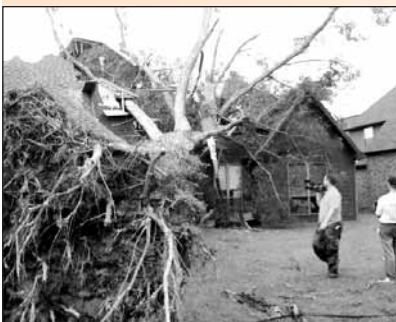
A twenty foot tree crashed through the roof of the home of RAI board member Woody Keim. Fortunately no one was in the room that was destroyed.
